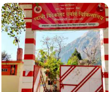
Pipalkoti, Shri Badrinath Marg, January 2018
